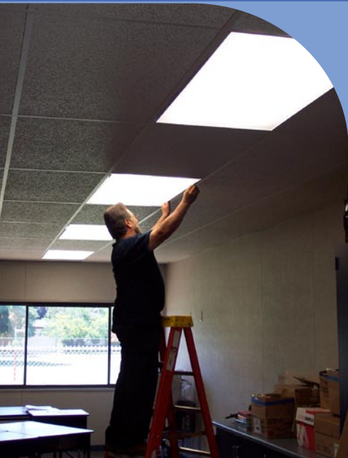
A contractor installs the new lamps at FUSD
