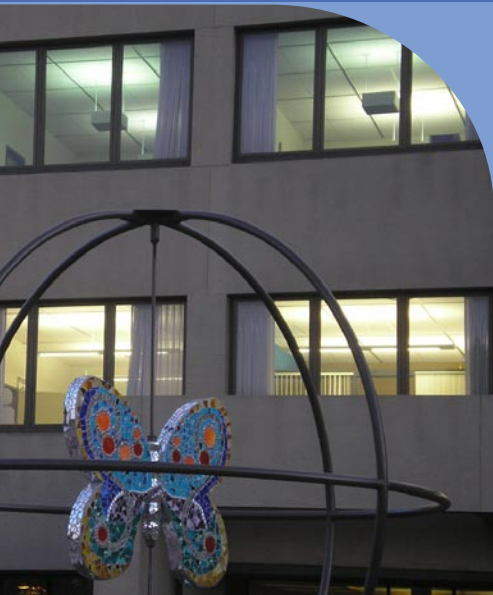
Before retrofit (upper floor) After retrofit (lower floor)
